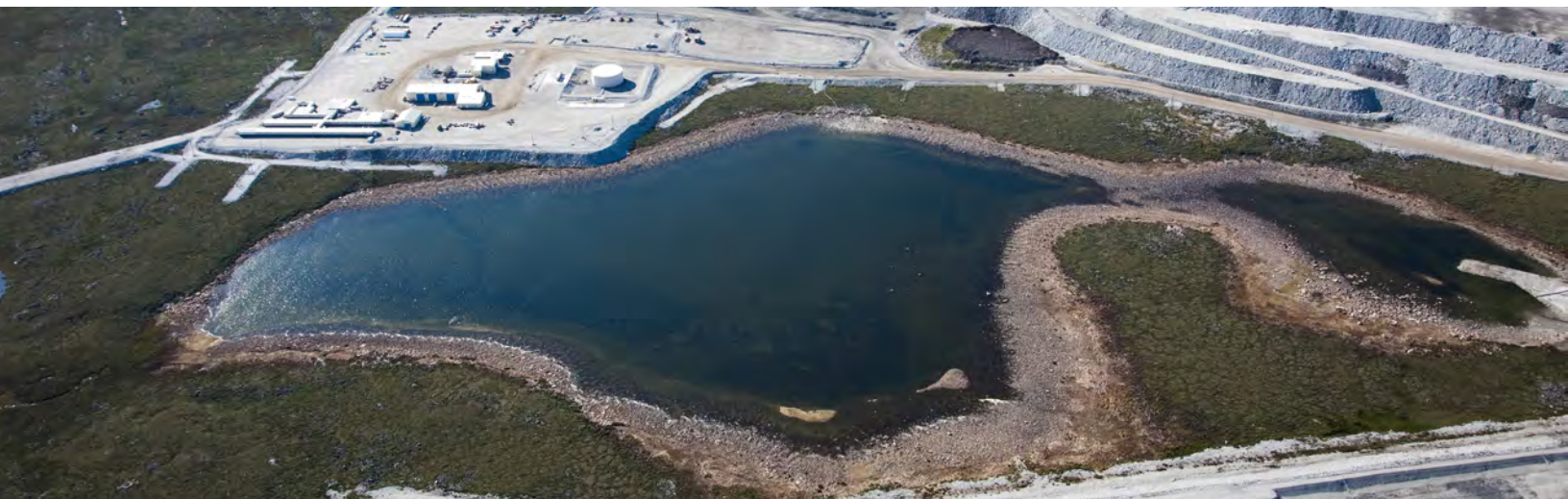
King Pond Settling Facility
