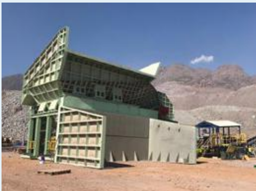
Construction is under way on the full-scale bulk-sorting site at El Soldado copper mine in Chile.
