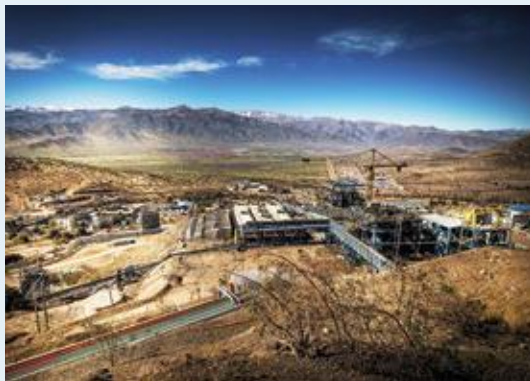
Las Tórtolas is a flotation plant, processing copper concentrate from the slurry pumped via a pipeline from Los Bronces mine, located 65 kilometres from Santiago and 3,500 metres above sea level. Los Bronces is one of the biggest copper mines in the world.
